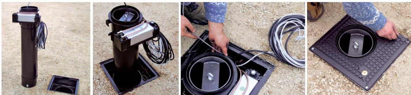
Installation operations: positioning the traffic control post inside the housing previously cemented into the ground, followed by electrical wiring and closure with a cover plate.
