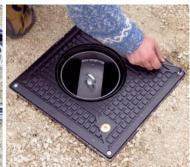
Installation operations: positioning the traffic control post inside the housing previously cemented into the ground, followed by electrical wiring and closure with a cover plate.
